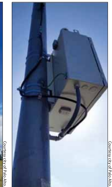
Palo Alto’s move to “advanced metering infrastructure” will require installation of five base stations with 10 boxes, like the one pictured on the right.
