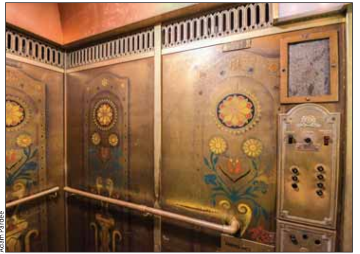
Stretched, painted leather adorns metal walls of an elevator at the President Hotel Apartments in Palo Alto on June 12.
