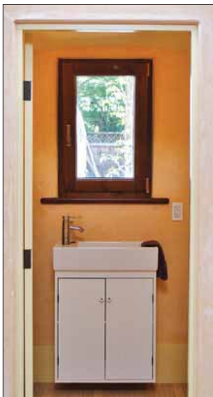
A very narrow bathroom sink hides wall plumbing for a future shower.
