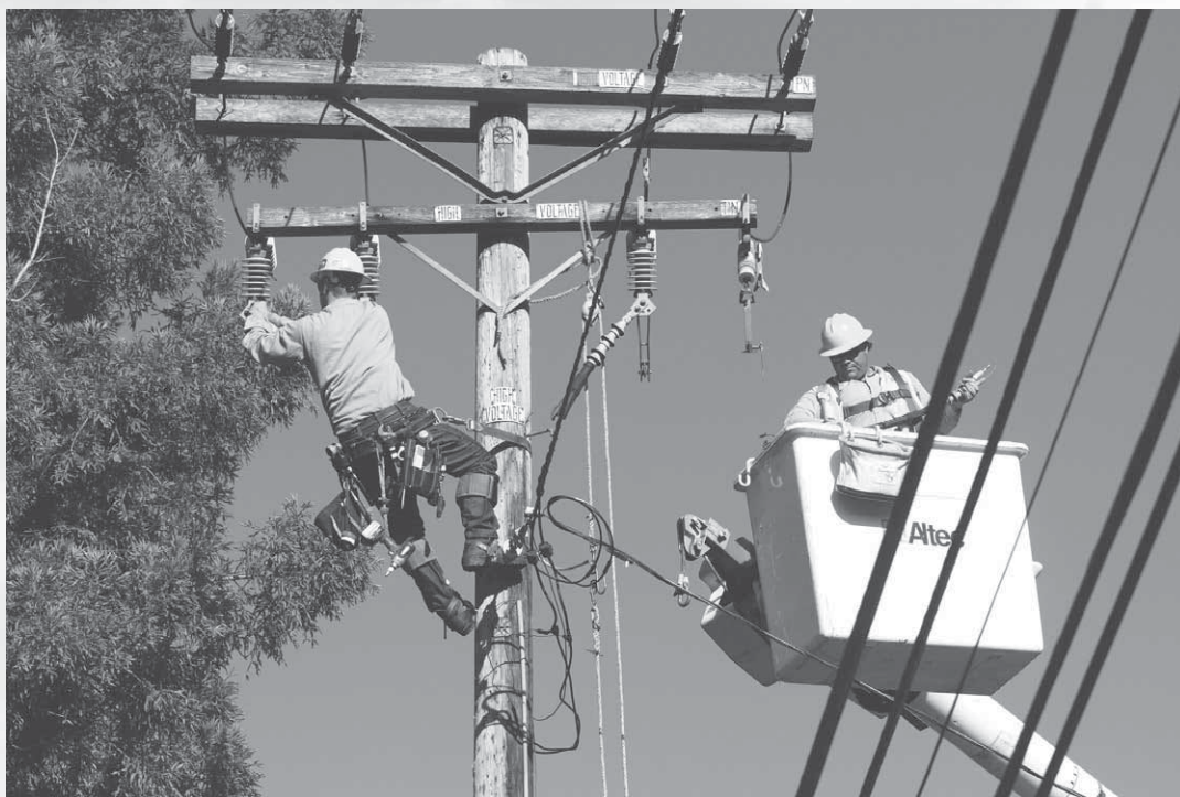
Palo Alto Utilities lineman apprentice Kevin Simpson, left, and lineman A.J. Santana replace a distribution power line on Coleridge Avenue on Jan. 8. In recent years the city has signed contracts with wind farms in Solano County.
