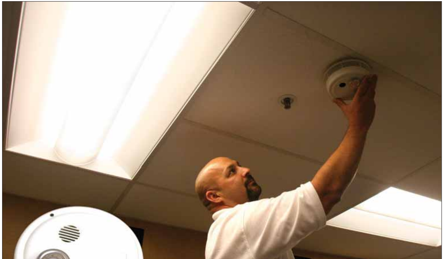
Photoelectric smoke detectors, like this one created by Gentex, left, have shown to be more effective than ionization alarms in detecting smoldering fires. Above, Frank "Mo" Miranda, fire systems supervisor at Stanford University, demonstrates how a photoelectric smoke alarm is installed in a ceiling at the Environmental Safety Facility.
