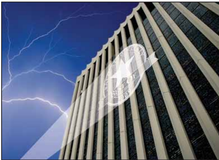
Palo Alto City Hall would be a great place to shine the Bat Light from, readers say.
