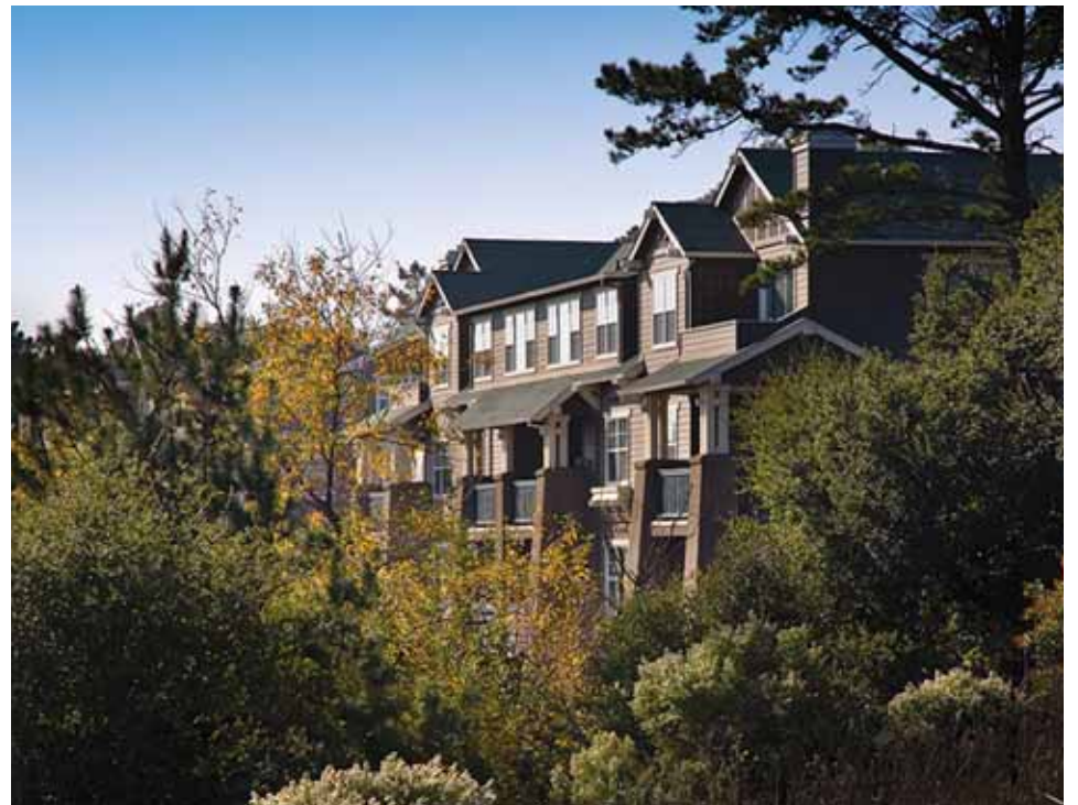
A 44-unit apartment complex called College Vista was opened in late 2004 for faculty and staff of the San Mateo Community College District. Offering rents at roughly half market rate, the district is attempting to prevent high staff turnover.
