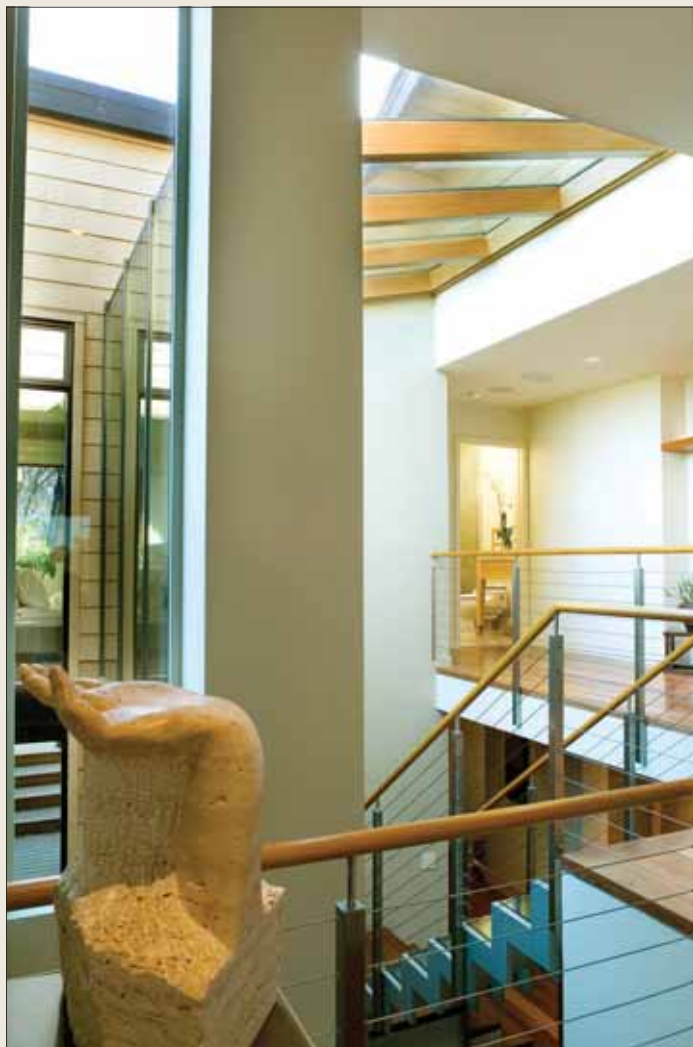
The floating staircase is made from one piece of solid steel, with glass treads and a stainless-steel rail.
