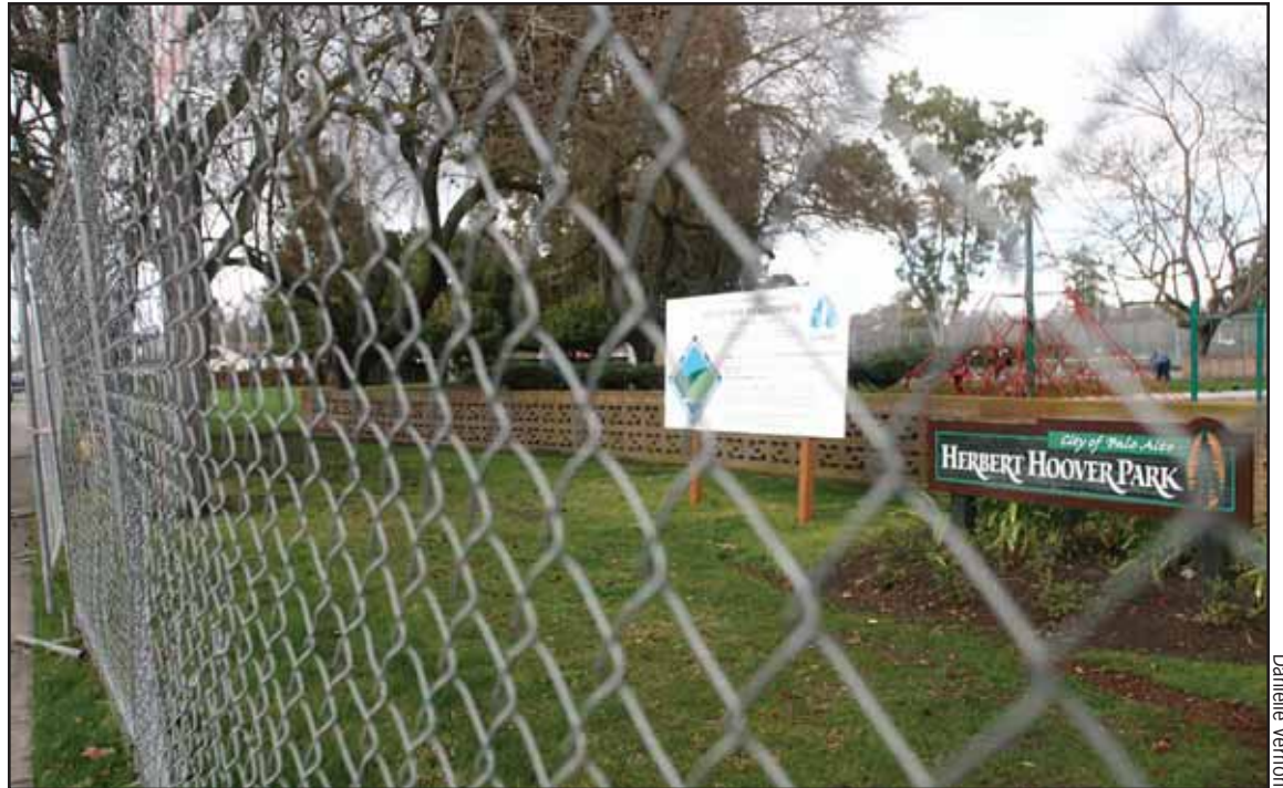
A public-private partnership between the city and Palo Alto Little League will revamp the Hoover Park infield.
